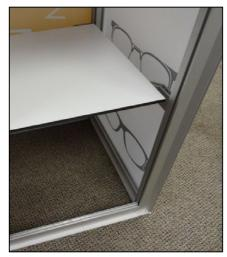
5. Install the optional counter shelf brackets to the corner posts. Set the shelf on the brackets.
