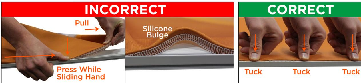
Pulling on the silicone welt during installation stretches the silicone and creates a bulge in the silicone welt that is difficult to correct smoothly.
